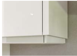
Feature wall end panel - the profile follows the return on the corner
